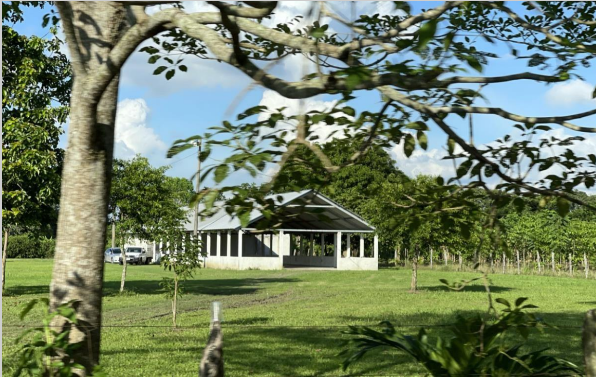
End view of camp pavilion
