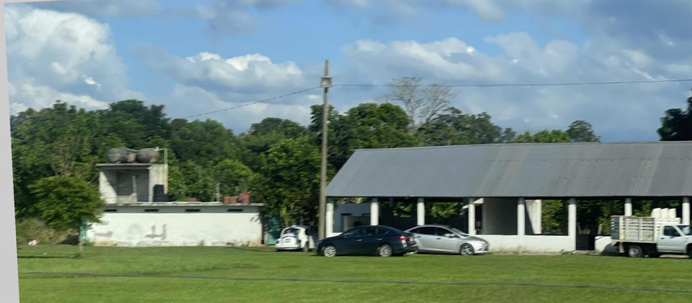
Side view of camp structure (kitchen left, open area to right)
